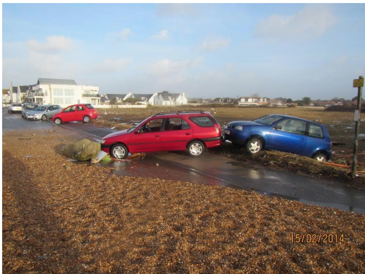
Figure 2-8: Photograph of damage caused by wave overtopping to the east of Hurst Road East car park in February 2014 (obtained from NFDC)
