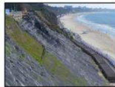
Cliff Slope Stabilisation
