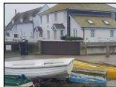
Deployable defences (e.g. flood gates)
