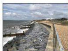
Rock Revetment / Armour
